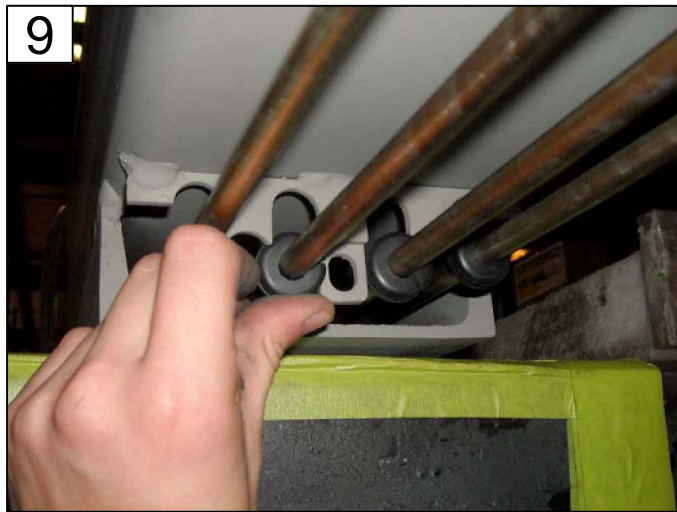
PUSH GROMMETS AROUND TUBES PAGE 15 - ITEM 15
